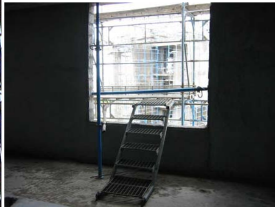
Proper Access to workplatform
