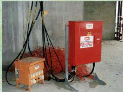
Rising Main Unit and Transformer
