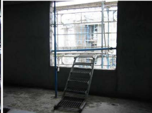
Proper Access to workplatform
