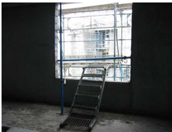
Proper Access to workplatform
